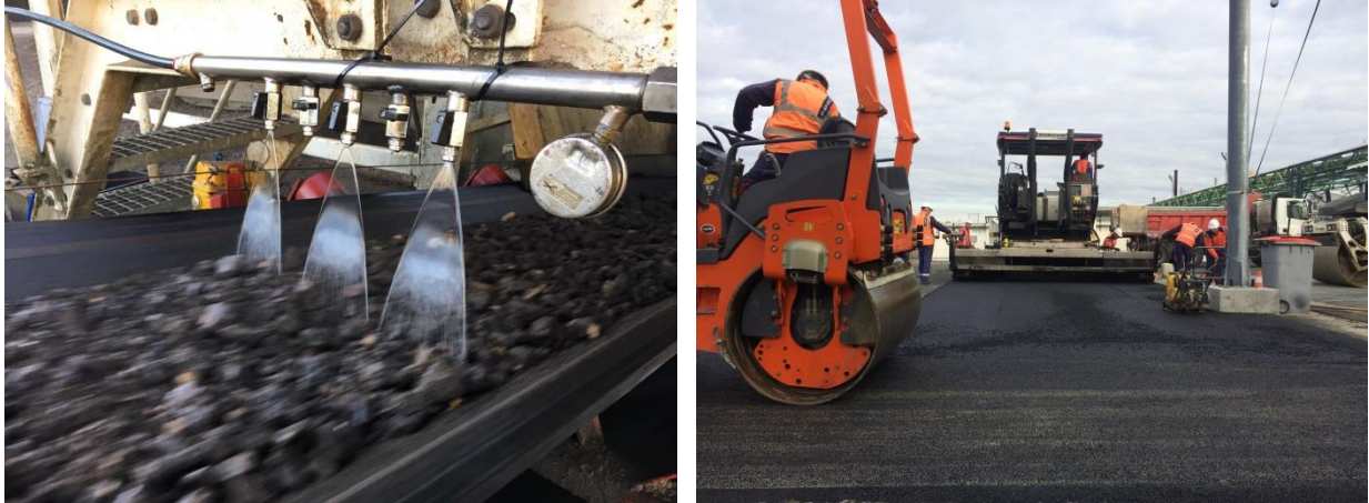
FIGURE 2. RA treated at the mix plant and job site application
