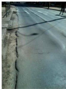
FIGURE 1: Rutting formed by the permanent deformation of the material (a) and non-structural deformation scheme of the asphalt layer (B) (author and adapted from [8])
