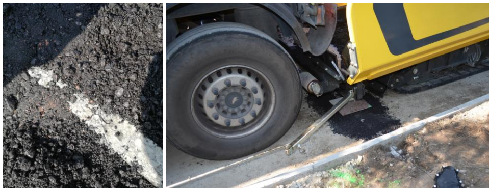
FIGURE 5 Installation of FBGs in base asphalt layer directly on the base
