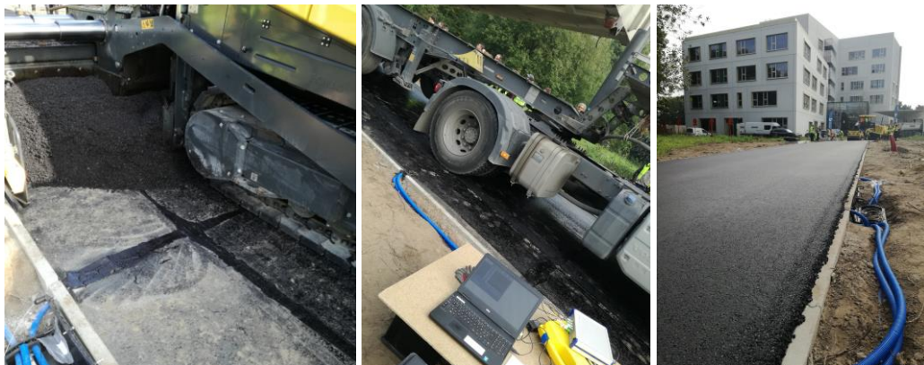
FIGURE 6 Installation of FBGs in two base layers
