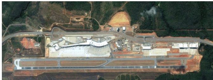
FIGURE 4 Tancredo Neves International Airport. Source: Google, 2017
